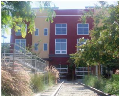
At the Santiago Street Lofts, located in Santa Ana, public transportation is immediately available.
